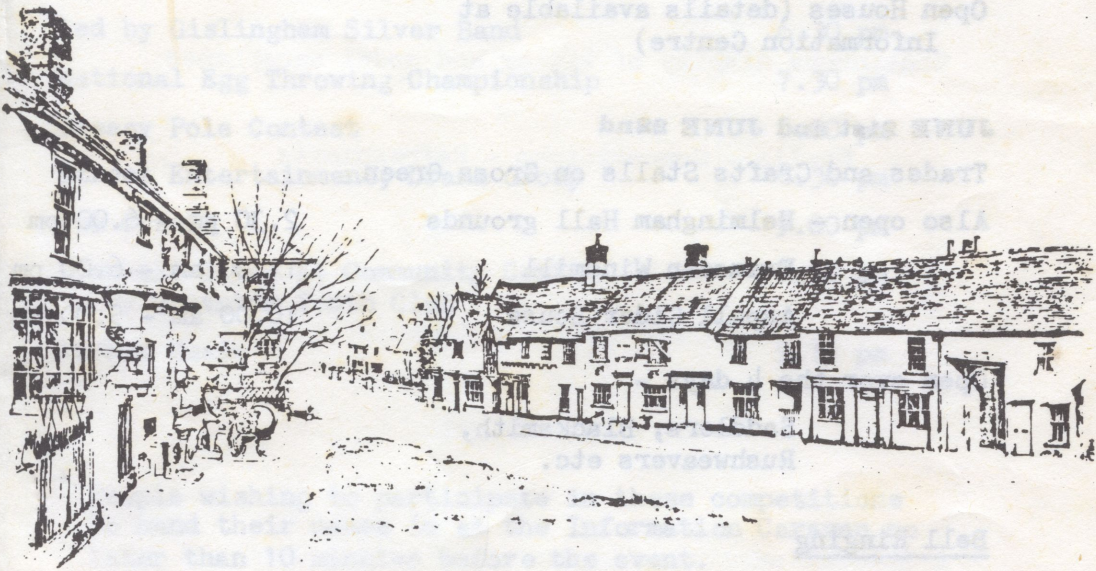
The high street Debenham Suffolk
