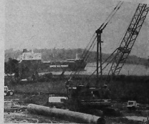
NOVEMBER 1979. The first stages of the bridge foundation
